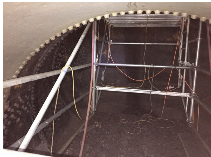
Fig. 9. Scaffolding set up inside the penstock.
