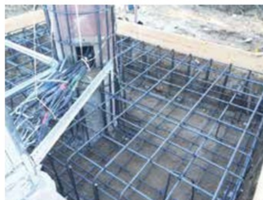
Figure 5. Foundation and the steel dowels at the base of the pole.
