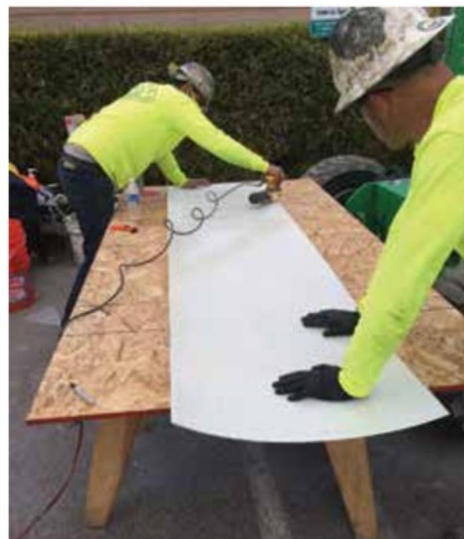
Figure 4. PileMedic laminates being cut to size on the job site before it is wrapped around the pole.
