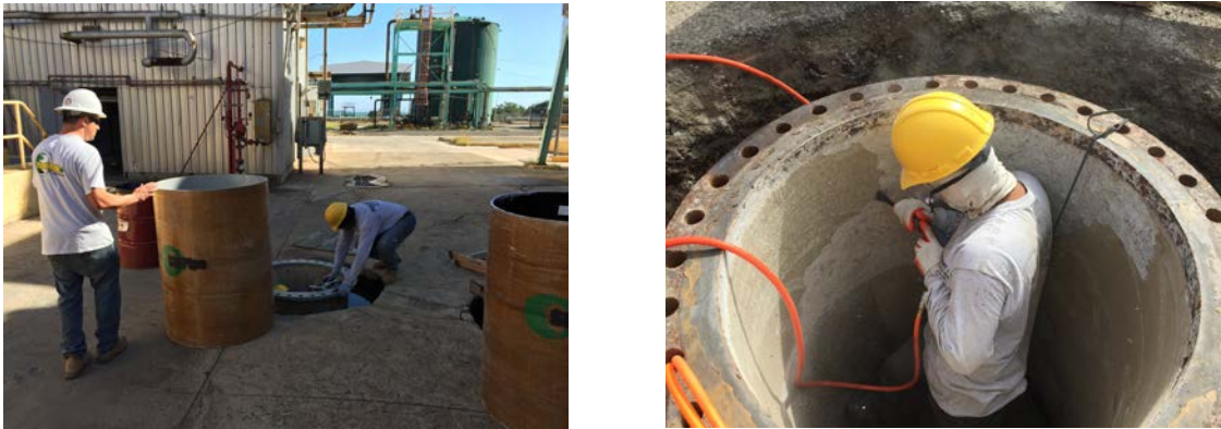
Fig. 7. PM carbon FRP pipe segments placed by riser pipe and removing laitance from the interior surface of the pipe.
