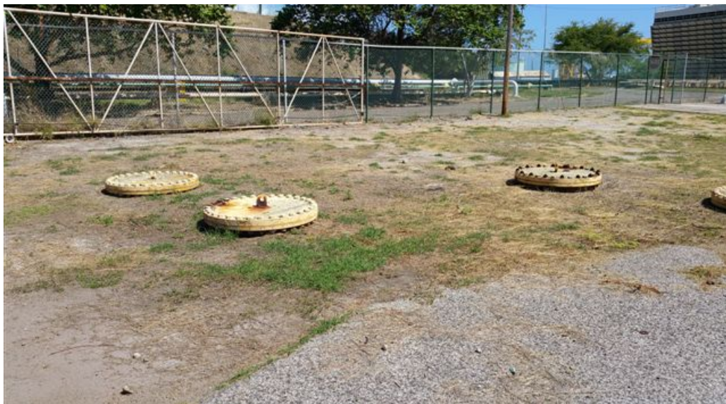
Fig. 2. Typical riser pipes with bolted lids throughout the power plant
