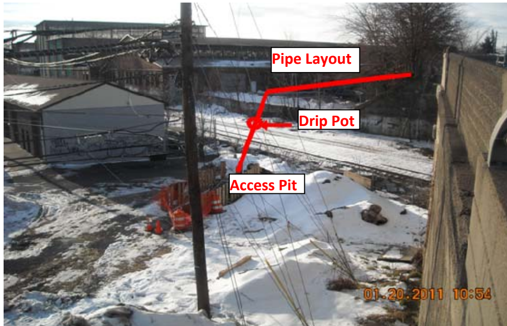
Figure 6. Project site showing the existing pipe layout and drip pot location under the railroad tracks.
