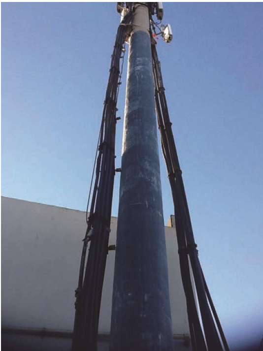
Fig. 4: Carbon and glass FRP applied to the lower 26 ft (7.9 m) of the pole
