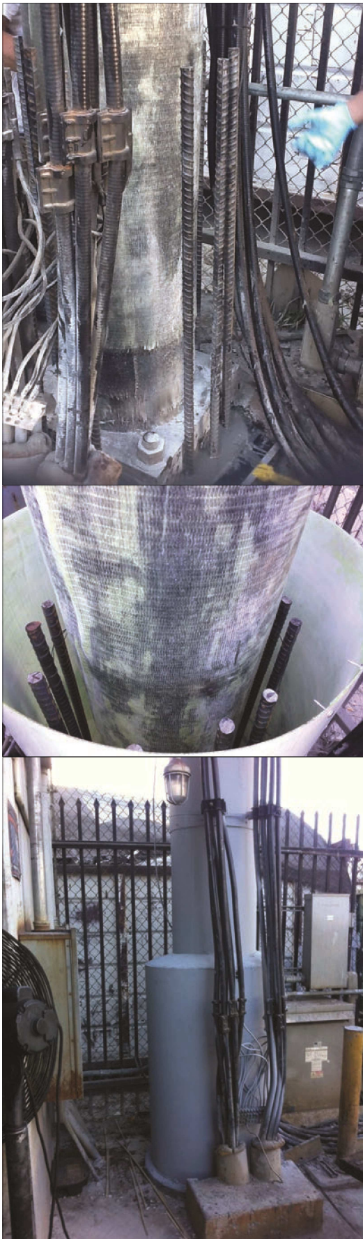
Fig. 6: Reinforcement detail near the base showing the anchored steel, FRP laminate shell, and the finished installation
