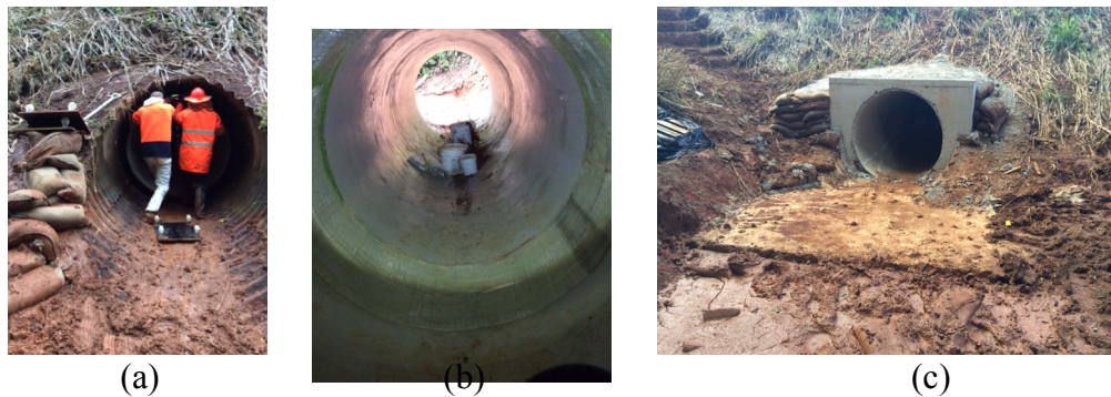
Fig. 4. (a) Caster trolleys inside the culvert allowed pushing lightweight StiffPipe® segments by hand into the culvert; (b) joining of segments with wet layup; (c) finished project
