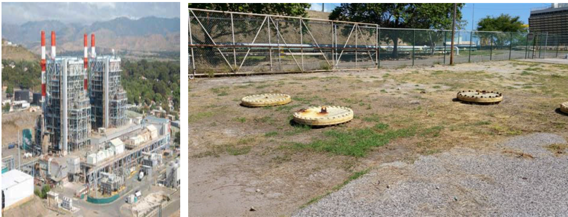
Fig. 5. Aerial view of Aguirre Power Plant (Salinas, PR) and typical pipe risers and lids
