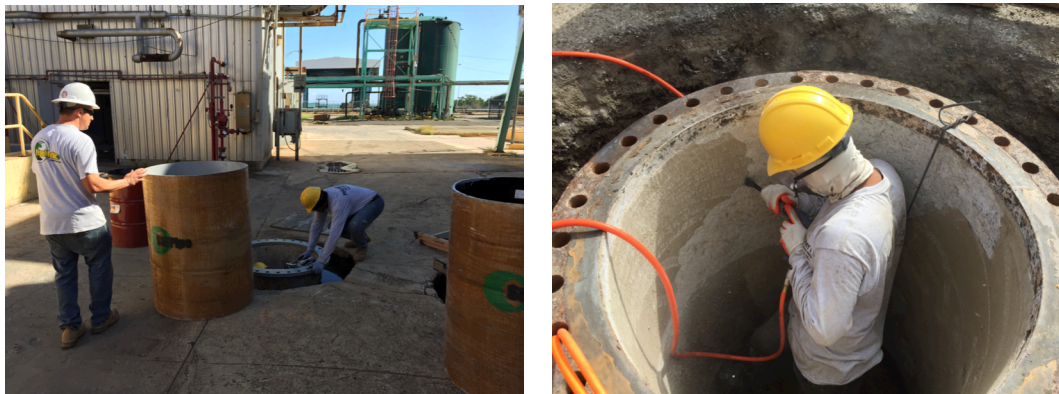
Fig .9. SC carbon FRP pipe segments placed by riser pipe and removing laitance from the interior surface of the pipe.
