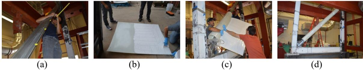
Figure 3. Retrofit for BRB using BraceWrap® includes: (a) applying debonding material, (b) apply epoxy, (c) wrap laminate around the brace to create a tube, and (d) fill the tube with concrete.
