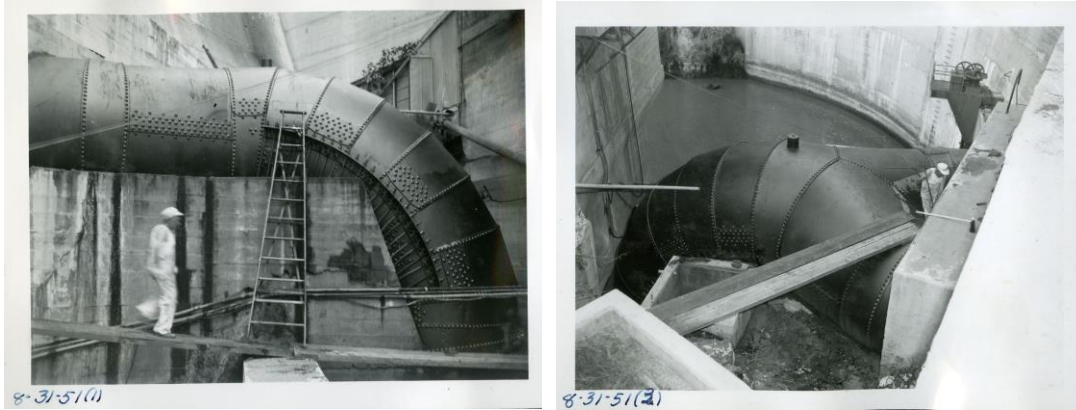
Fig. 3. Periodic inspection and maintenance of the exterior of the penstock – circa 1951.
