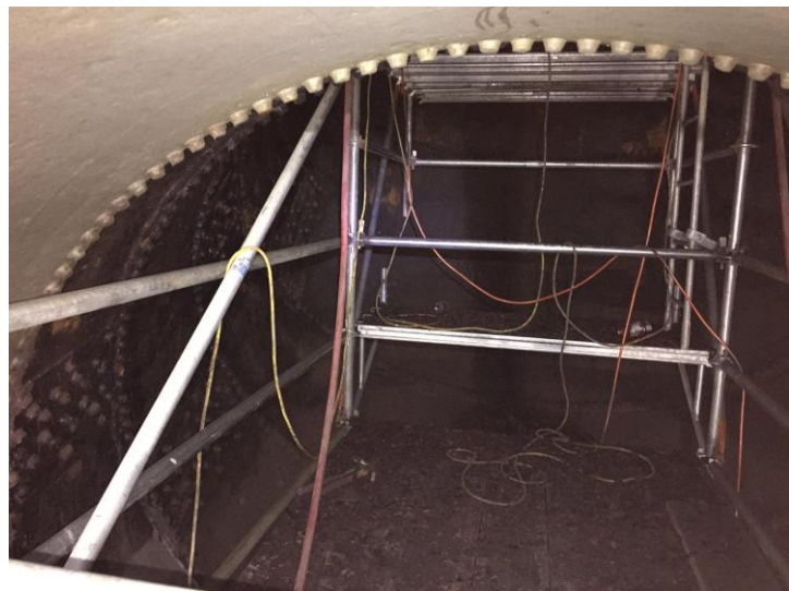
Fig. 9. Scaffolding set up inside the penstock.
