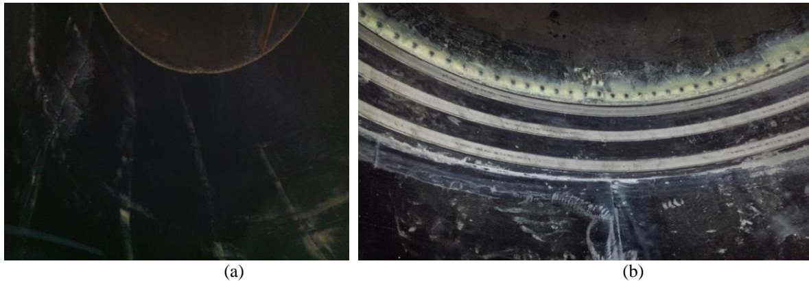
Fig. 11. (a) Repaired penstock prior to application of topcoat and (b) at termination point showing Weko Seal
