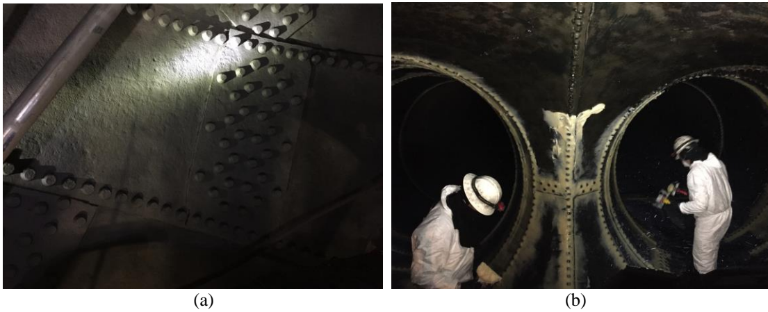
Fig. 10. (a) close-up of the rivets inside the pipe and (b) coating the rivets with thickened epoxy.
