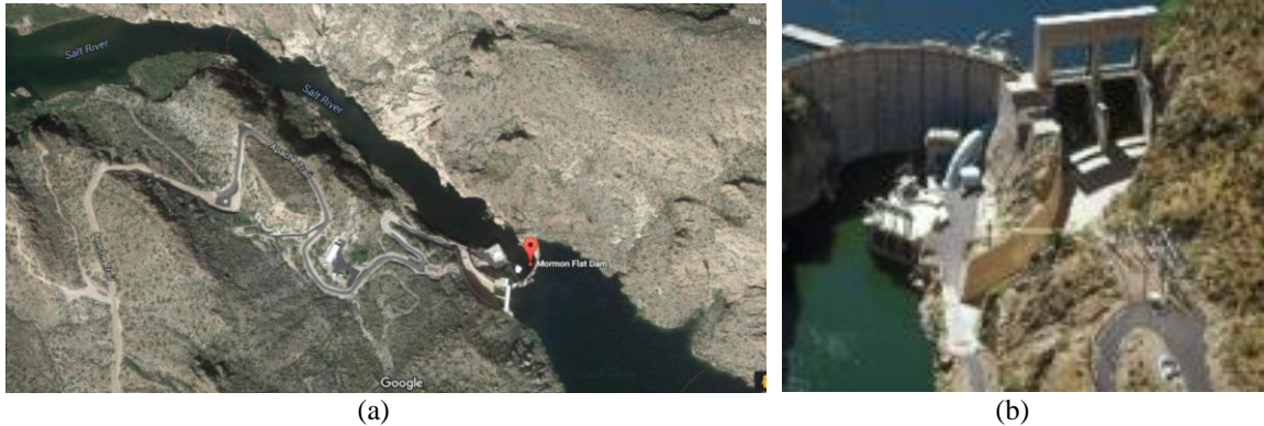
Fig. 4. Limited access to the dam: (a) through a winding road and (b): a small parking area.
