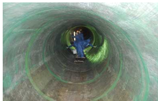
Figure 5: Installation of FRP sheets on the interior surface of the pipeline.
