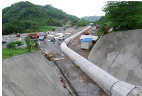
Figure 1: Above ground segment of the “El Encanto” pipeline
