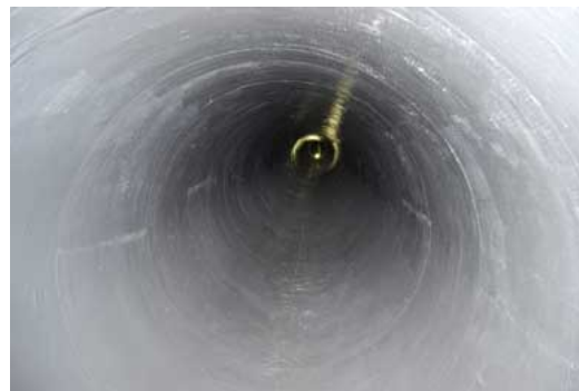
Figure 6: Completed segment of pipeline prior to testing.
