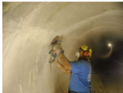
Figure 4: Prep work prior to installation of FRP lining
