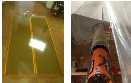
Figure 5. LaminaHeat and propane heater tried in curing the pipe.
