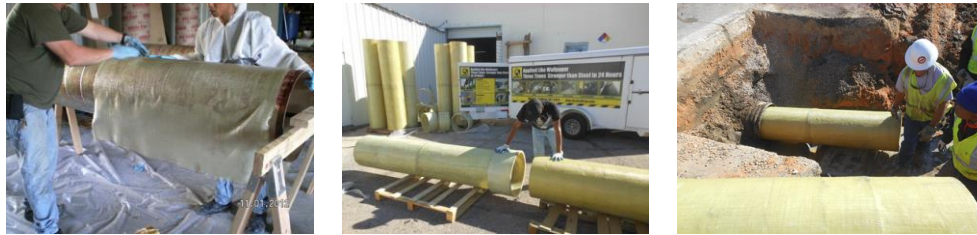
Figure 1. Honeycomb-FRP pipe being made on a mandrel for repair of culvert.
