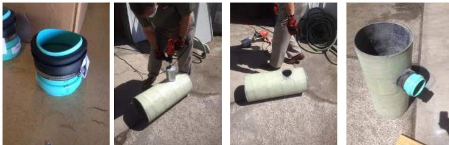
Figure 6. Installation onto InfnitPipe ® of a lateral connection made by Inserta Tee ®
