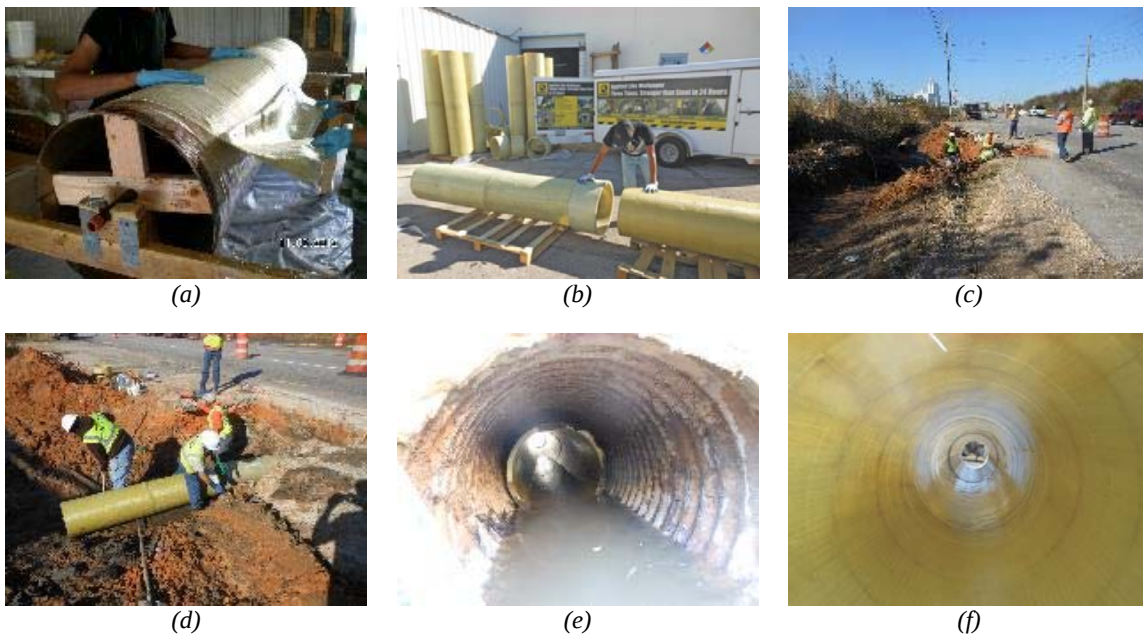
Fig. 8. Slip-lining a corroded culvert in Mobile, Alabama with StifPipe®: (a) glass fabric layers wrapped around the mandrel, (b) manufactured pipe segments prior to shipment, (c) view of the job site, (d) light-weight pipes being connected and slipped into the culvert by hand, (e) culvert partially slipped, and (f) finished repair
