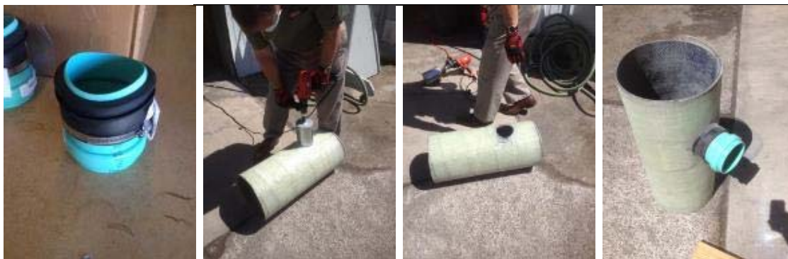
Fig. 10. Installation onto InfinitPipe® of a lateral connection made by Inserta Tee®
