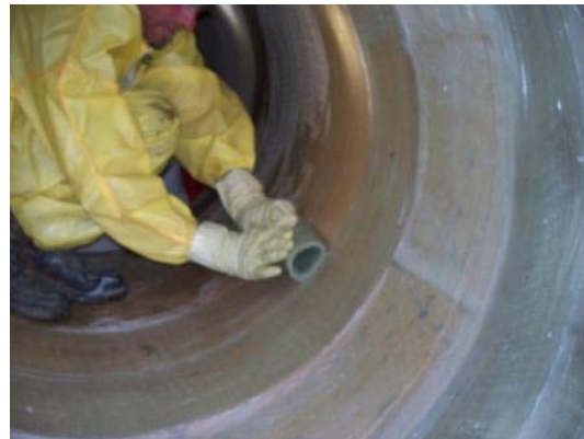
Figure 1. Repair of pipes with wet layup FRP
