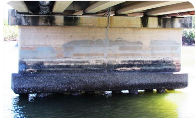
Figure 1 - View of typical pier
