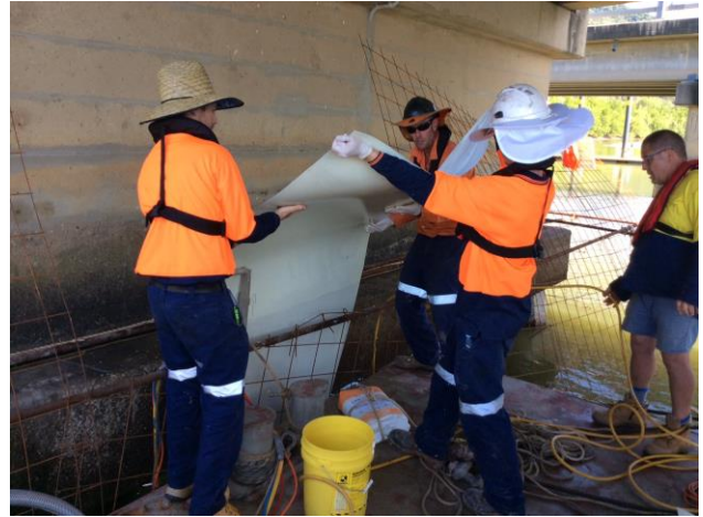
Figure 12 - Laminate being passed to the diving crew for installation
