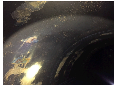
Fig. 3. Damaged tar coating and internal corrosion of pipe
