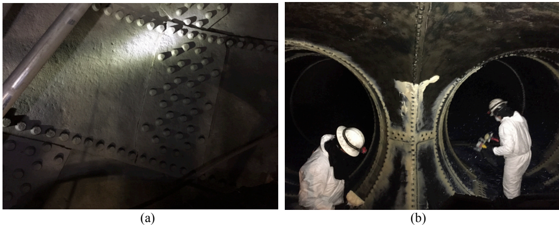
Fig. 10. (a) close-up of the rivets inside the pipe and (b) coating the rivets with
