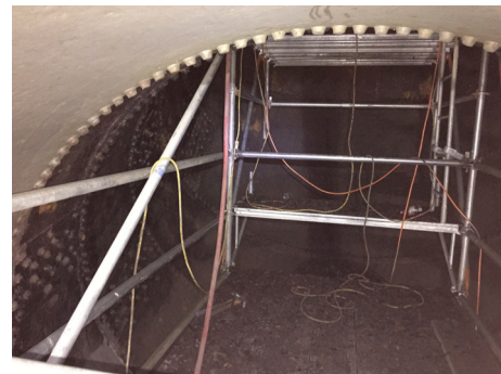
Fig. 9. Scaffolding set up inside the penstock.
