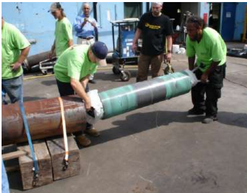
Figure 6. Insertion into pipe section.
