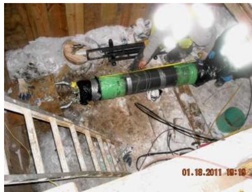
Figure 19. Inflatable pig/laminate being inserted.
