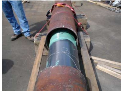
Figure 7. Laminate in position and pig being inflated.
