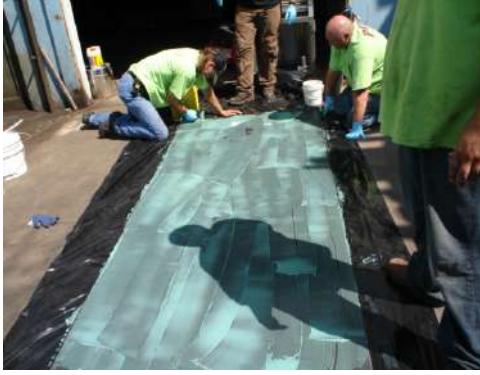
Figure 4. Adhesive application.
