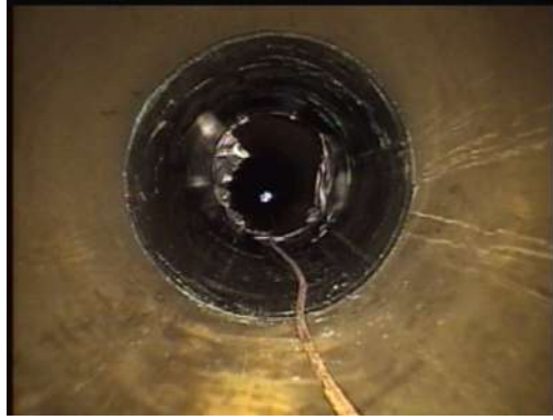
Figure 20. Final drip pot bridge laminate assembly.
