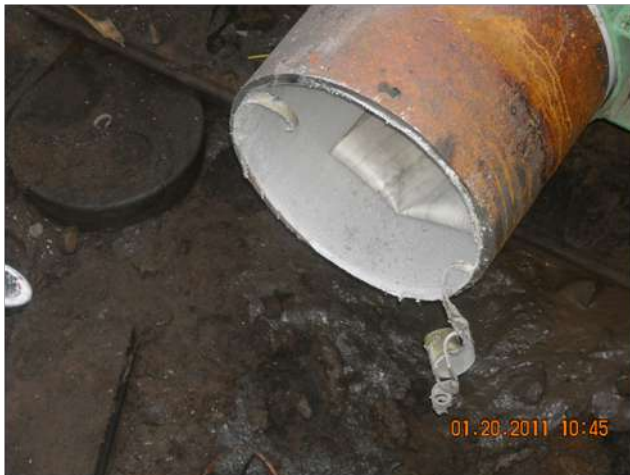
Figure 21. Excess liner being trimmed at pipe-ends.
