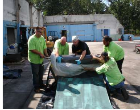
Figure 5. Laminate installed onto inflatable pig.
