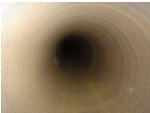
Figure 18. Pipeline ID fully cleaned.
