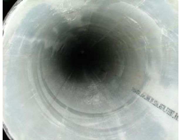
Figure 22. Completed liner installation with the FRP laminate
