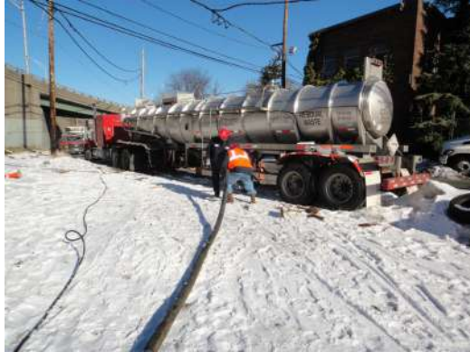
Figure 16. Equipment utilized for water jetting operation.
