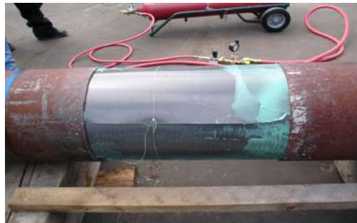
Figure 8. Final installation in simulated drip pot.
