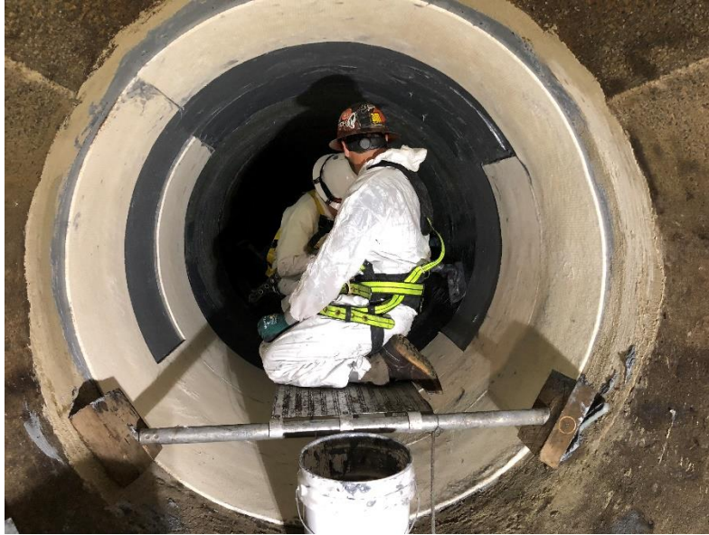
Figure 8. Installation of the FRP with the 3D core sandwich structure (StifPipe®) with the wet layup method 1 .
