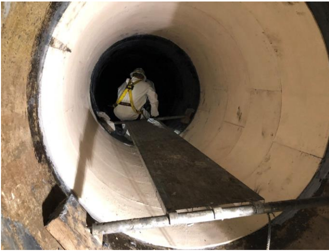
Figure 3. Installation of .57 in. thick StifPipe® inside the 66-inch RCP.
