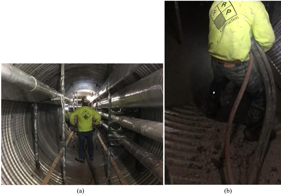
Fig. 5. (a): Attachment of steel wire mesh; and (b) application of gunite.
