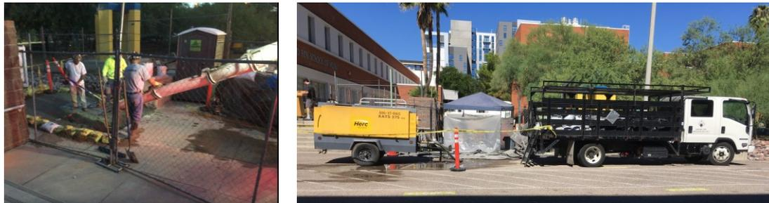
Fig. 8. Placement of concrete to restore the collapsed sidewalk area
