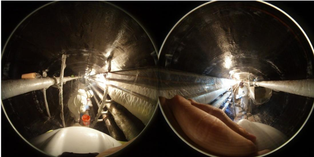
Fig. 6. 360-degree view of the tunnel looking forward and backward during the installation of the FRP.
