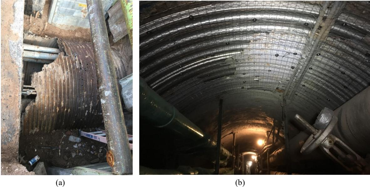
Fig. 3. (a): Removal of the soil above the failed tunnel and shoring of the trench; and (b): Placement of new corrugated segment at the crown and the steel reinforcing wire mesh.
