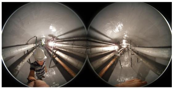
Fig. 7. 360-degree view of the tunnel looking forward and backward during the final inspection after the installation of the FRP and top coating.
