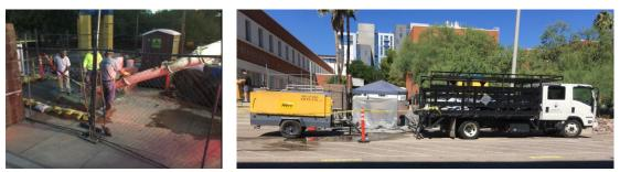
Fig. 8. Placement of concrete to restore the collapsed sidewalk area
