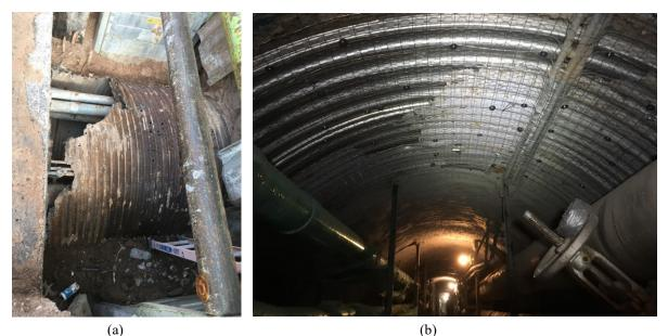
Fig. 3. (a): Removal of the soil above the failed tunnel and shoring of the trench; and (b): Placement of new corruga segment at the crown and the steel reinforcing wire mesh.
