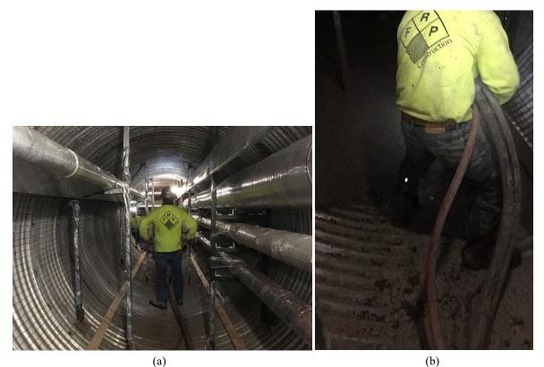
Fig. 5. (a): Attachment of steel wire mesh; and (b) application of gunite.
